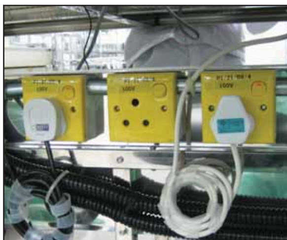
Power Strip Mounting Panel
